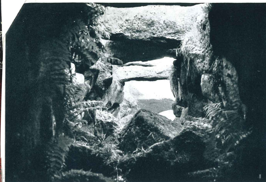
'The Earth House,' called by the St. Kildans 'the fairy house,' is a long underground dwelling, roofed across the narrow passageway with huge lintel stones
